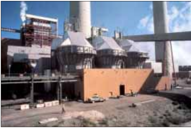
Figure 1 Jim Bridger Power Station with sodium carbonate scrubbers installed by B&W.
